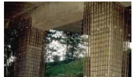
Structural strengthening with Emaco Nanocrete R4 Fluid.
