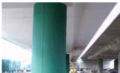
Masterseal: 136 / 138 / 190 coatings limit the oxygen transport through the concrete.
