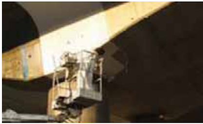
Principle 1, method 1.2 Masterseal protective coatings: Available as rigid, flexible, acrylic, EP or PU material, protect against all kinds of ingress.
