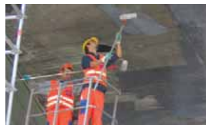
Hydrophobic treatment using Masterseal 303.
