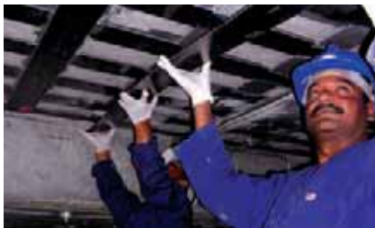
Principle 4, method 4.3 MBrace structural strengthening: Glass, carbon, aramid based.
