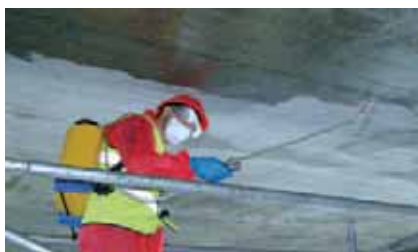
Corrosion at the cathodic areas of the reinforcement is inhibited by the use of Protectosil CIT.
