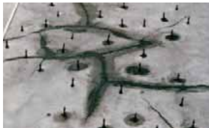
Concessive injection products: Used for force transmitting filling (load transfer) of cracks.
