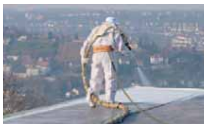
Conipur waterproofing systems: Eliminate water penetration and allow the concrete to dry out.
