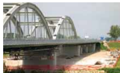
Masterseal coatings applied directly on the concrete to protect the underlying reinforcement.
